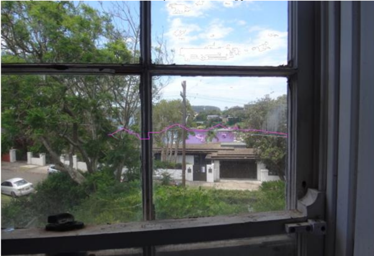
The image below is from the 1 st floor secondary bedroom - standing position
